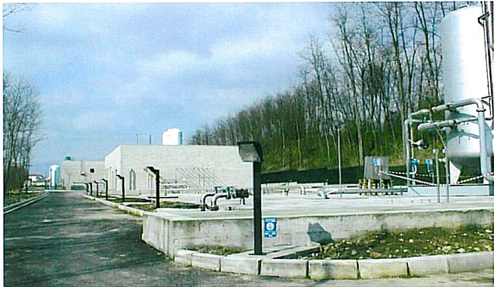
7 – COLOR AND SURFACTANT REMOVAL AT ALTOURA; 80 KgO 2 /h AND 1.000 m 3 /h CAPACITY
