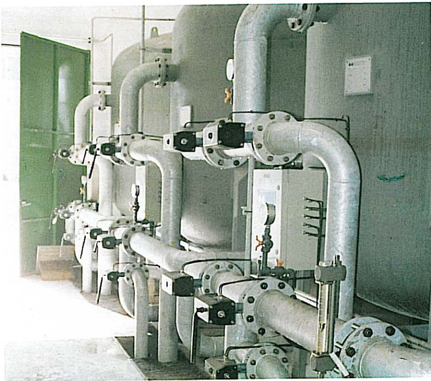
16 - DRINKING WATER PLANT
