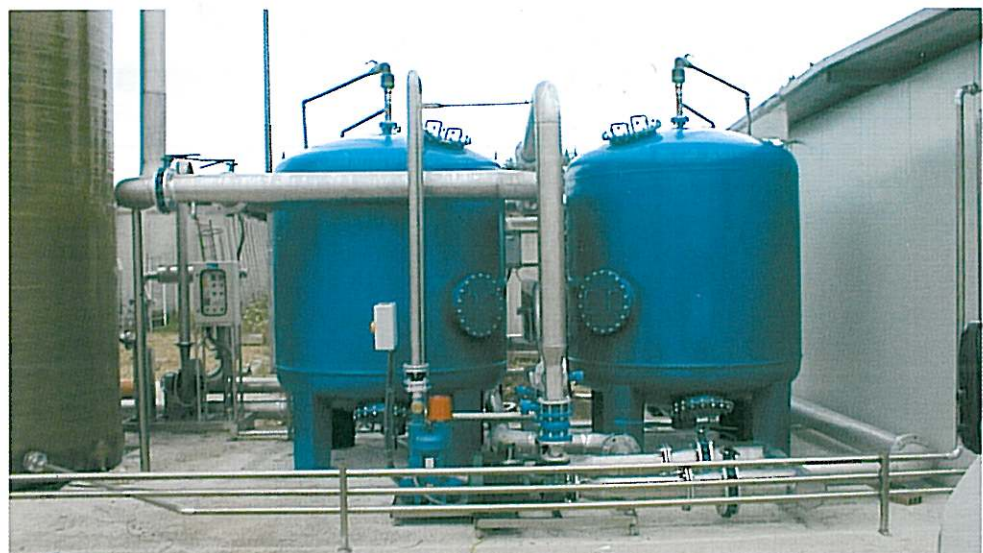
9 – IRON AND MANGANESE REMOVAL PLANT
